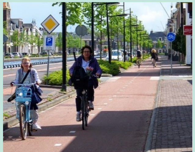
Exhibit 2: A well integrated street with walking path, step-separated bicycle lane, and parking
