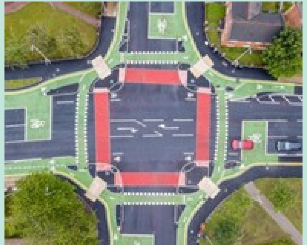
Exhibit 6: A Cycle Optimised Protected Signals (CYCLOPS) junction in Hulme, Manchester, maximizes opportunities for safer cycling and walking
